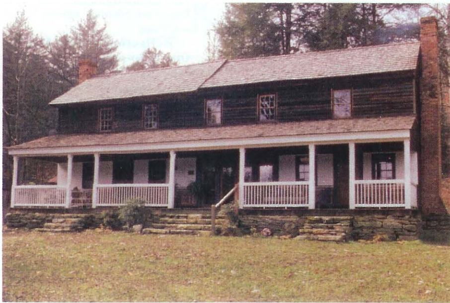
Back to life. When Arthur and Zee Campbell purchased the c. 1826 Albertus Ledbetter House near Marion, N.C., the structure’s foundation had sunk and the house appeared beyond repair. Now this rare surviving example of transitional Federal/Greek Revival architecture and post-and-beam construction looks just as it did more than 150 years ago.
